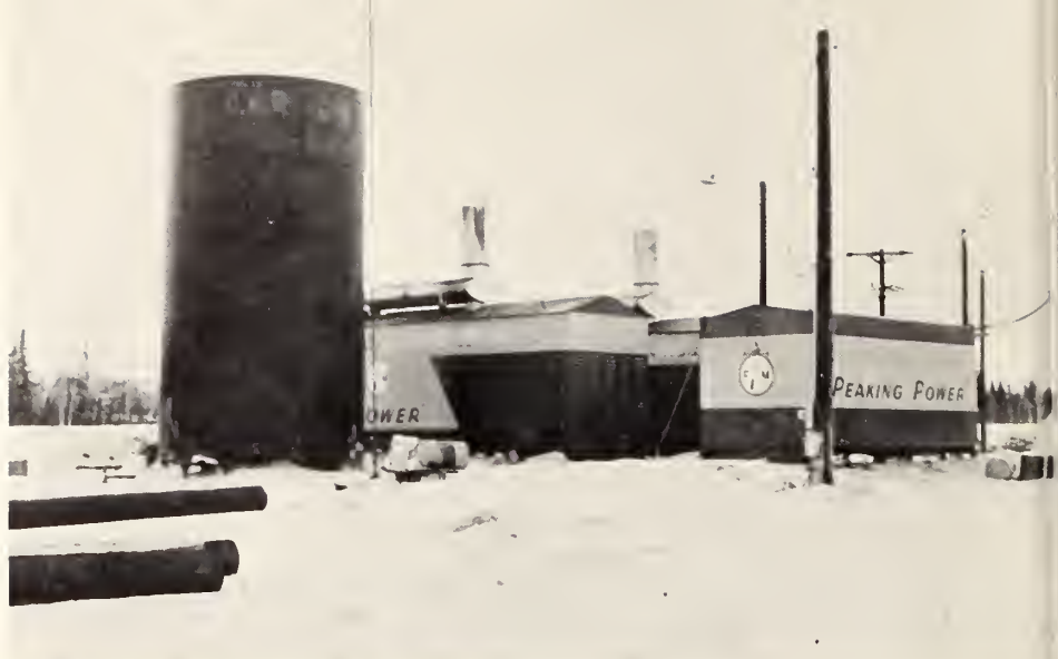
Packaged diesel units, right, or gas turbines, below, are used to generate power in remote Alaskan villages. Isolation and extreme weather conditions make long-distance transmission lines impractical.
